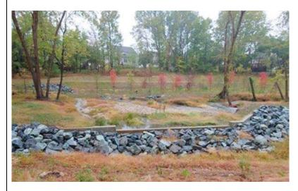
*Project 2:* The Plaza Drive Stormwater Pond Retrofit to Submerged Gravel Wetland, completed in Fall of 2018, provides treatment for 20.47 acres ISA.
