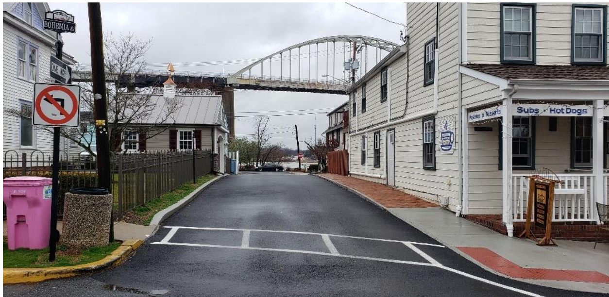
First Steet (West) New brick sidewalk with granite curbing, (Note: community recycling )
