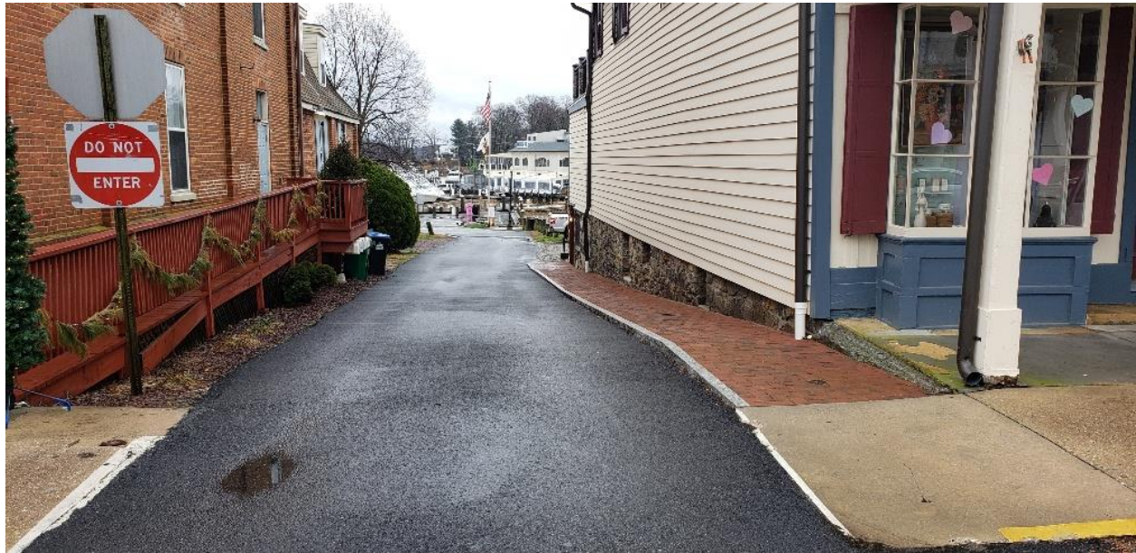
First Steet (East) – New brick sidewalk with granite curbing, and paving
