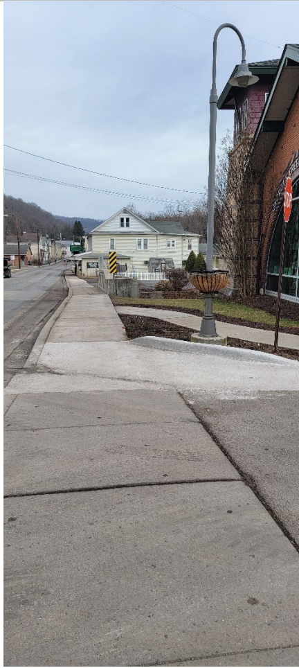
replaced curbing in front of library along Main Street
