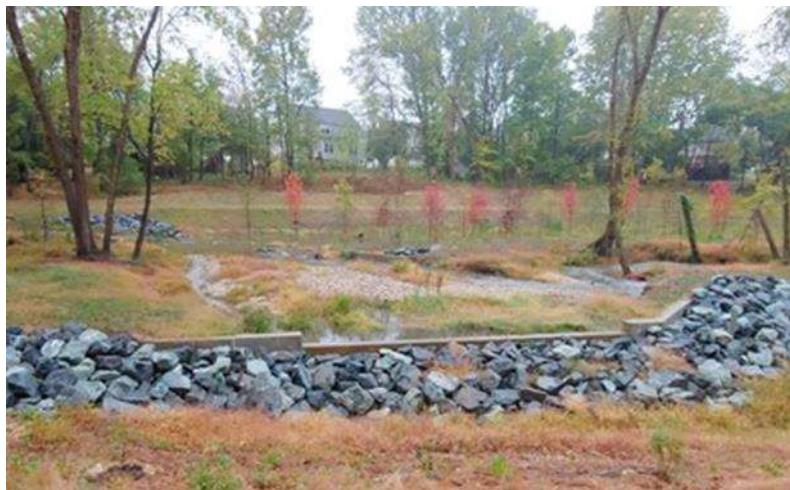
**Project 2:** The Plaza Drive Stormwater Pond Retrofit to Submerged Gravel Wetland, completed in Fall of 2018, provides treatment for 20.47 acres ISA.
