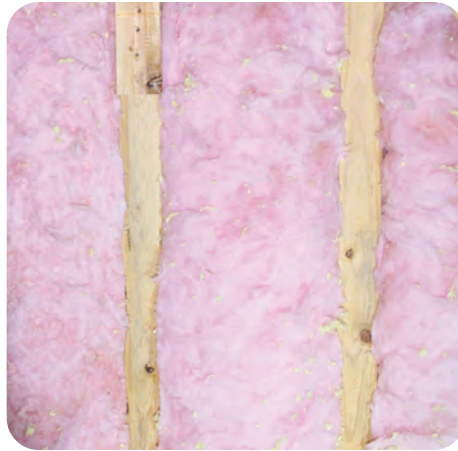
2. Cut batts for exact fit
