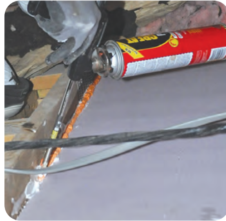
B-2. Seal around infill materials
