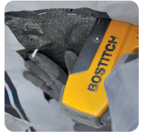
7. Stitch staple patch to ensure permanent adhesion
