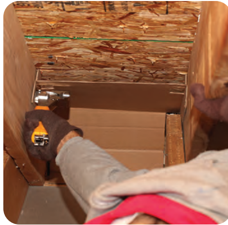
4. Install baffles, if needed. Ensure 2 inches of gap for airflow
