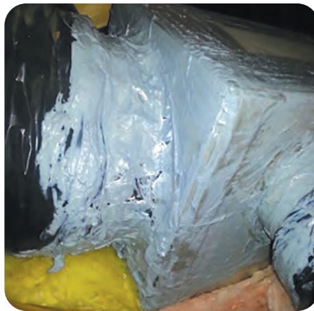
4. Seal new joints
