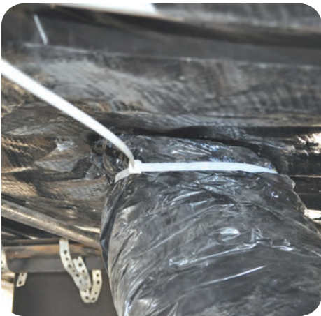
3. Secure vapor retarder layer at boots
