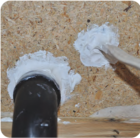
1. Ensure air sealing is complete
