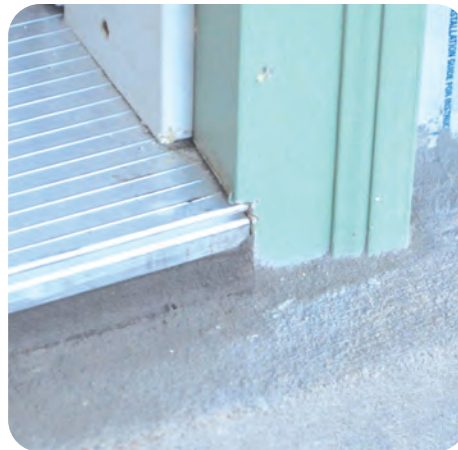
11. Seal along threshold, ensuring water will flow away from door
