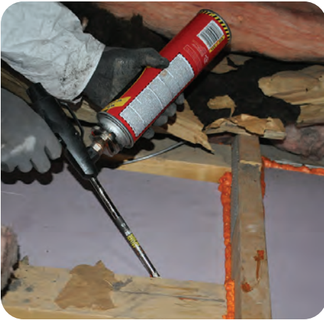
3. Ensure air sealing, if any, is completed
