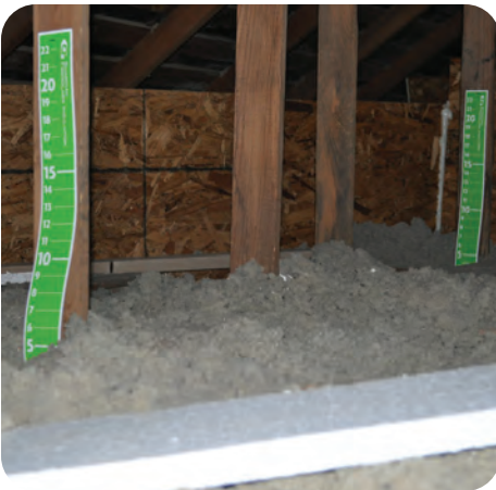
5. Depth rulers installed, 1 per 300 square feet
