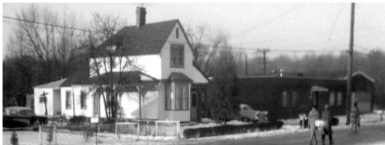
Figure 14. The intersection of Rhode Island Avenue, Lakeland Road and Navahoe Street was the social hub of Lakeland, with Black’s grocery store and soda fountain, a beauty parlor, the Elks Home and Lakeland Hall the focal points. All were destroyed during urban renewal. (Lakeland Community Heritage Project)
