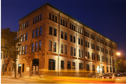
Miller's Court mixed-use rehabilitation in Baltimore
